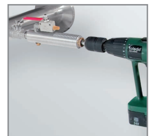
Drilling under pressure with CS drilling jig
